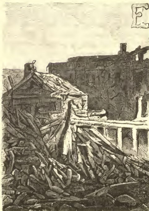
AFTER THE EARTHQUAKE.
